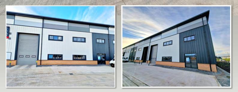
High bays with 8.5m to internal eaves / 10m to ridge
